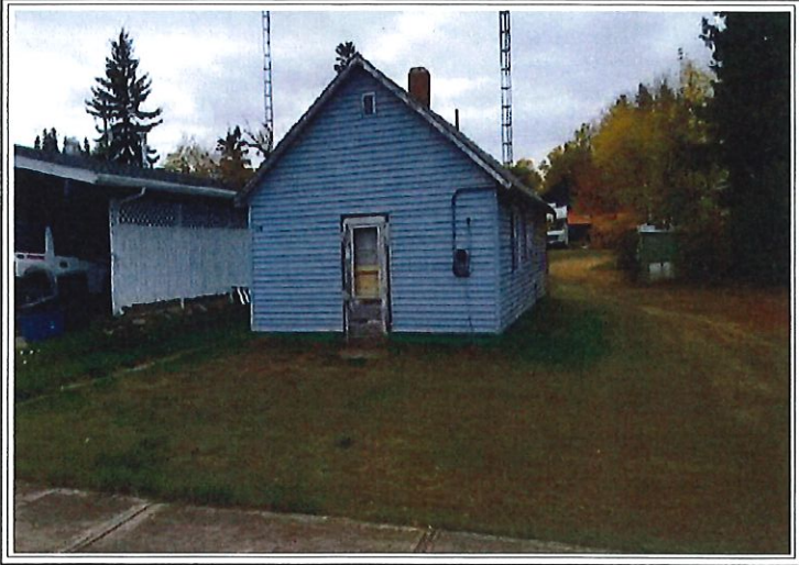
FRONT VIEW OF SUBJECT PROPERTY
